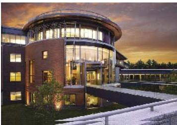
Blue Cross Blue Shield south shore headquarters
