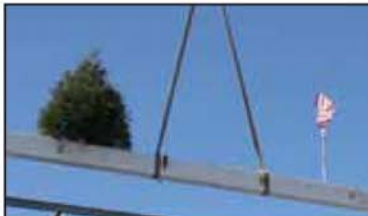
Hoisting the beam with the traditional pine tree and American flag
