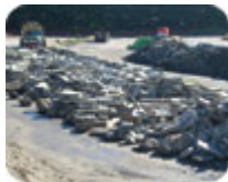
Granite curbing and asphalt were stockpiled to be crushed and reused.
