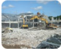
The existing concrete building was demolished with large excavators.
